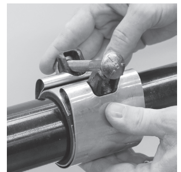
Drop in the bolt and tighten.
